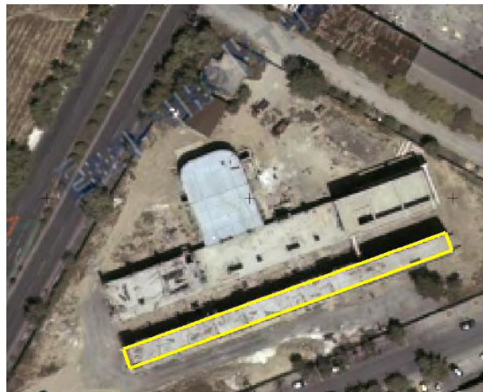
Fig. 3.1: Rooftop area of 400 m 2 , suitable for solar panel installation (photo and measurements taken from the national land registry of Greece) [59].
